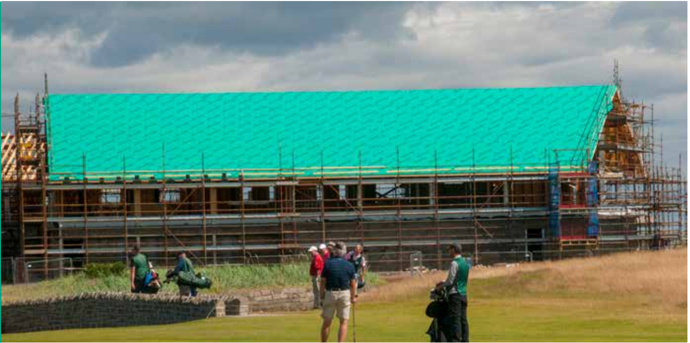
Carnoustie Golf Club Refurbishment
