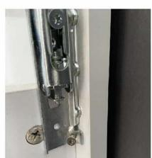
1. Locate and insert the Mounting Bracket (if not already in place). Make sure the Hanger is facing the wall side as displayed in the second image. Once in position, fix the Mounting Bracket with screw(already provided) to secure the Mounting Bracket as shown in the third image.
