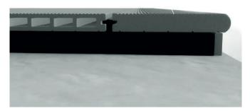
Step 4, once the bullnose board is in place and the fascia secure you can then admire your work. Dont forget to finish off hollow ends of decking with an end cap or corner trim. For information on how to install the rest of the decking, please visit our website.
