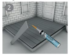
To fit the skirting trim you can either glue this using sumo grip adhesive or the trims can be screwed into the joists (Please note this method may cause the natural fibres to split) We advise the sumo grip adhesive option.
