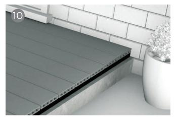
The ends of boards must be fully supported. No overhang or cantilever is allowed.
