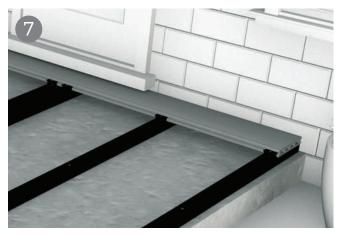
Our WPC boards are easily fastened to the joists of a supporting substructure with the help of our stainless steel screw and plastic T-Clip system. Start at the outside of the area to be decked. Place your first board and fix it to each joist it crosses using a row of starter clips.
