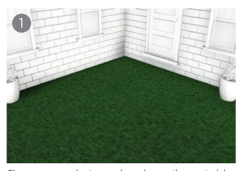
Clear away any plants, weeds, rocks, or other material that might be obstructing your site. Cut away the turf of the lawn by using an edger to cut the area and then a spade to remove it. Make sure the ground is level, you can do this by checking your site with a spirit level.
