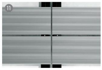
At butt joints - where the ends of two decking boards meet, this may mean doubling up on supporting joists as you will need to ensure that each board is held in place with it's own T-Clip where they meet.
