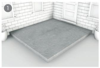
Make sure that the area to be decked is flat and stable. The concrete base should be at least **10cm thick** and have a slight slope - we suggest **a gradient of 1 in 80** - that runs away from the property to allow for the run-off of water that collects under the deck.
