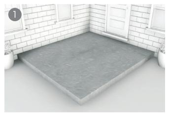
Step 1, Structural joists can be laid on top of a solid concrete base or a level area with weed mat covering. Make sure that the area to be installed on is flat and stable. If using a concrete base it should be at least 10cm thick and have a slight slope – we suggest a gradient of 1 in 80 – that runs away from the property to allow for the run-off of water that collects under the deck.
