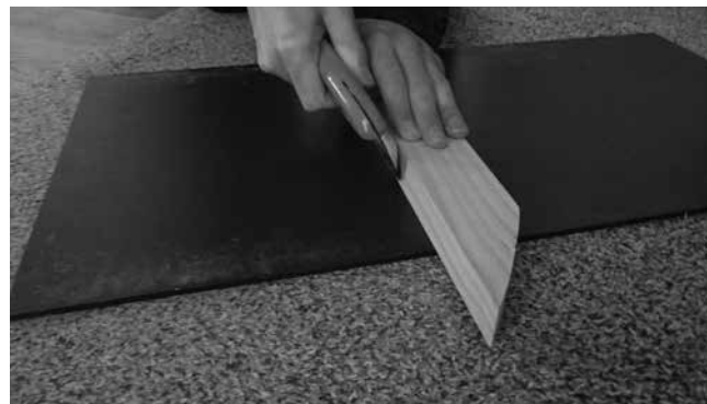
Fig. 2 – Cutting fibre cement slate using a scriber
