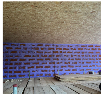
Passive Purple Passivhaus Airtight Sealant applied to wood fibre.
