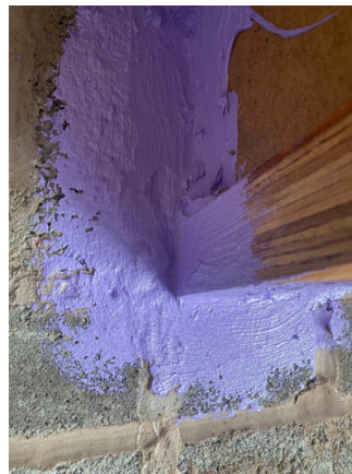
Joist connection on to masonry wall.
