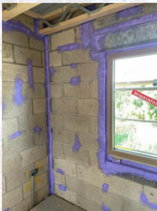
Internal brick connections.
