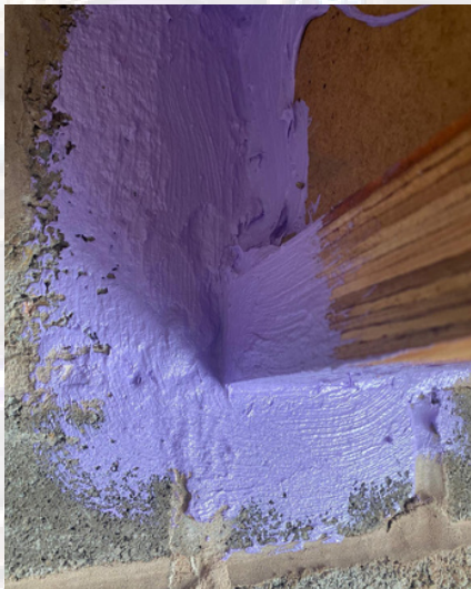
Joist connection into masonry wall
