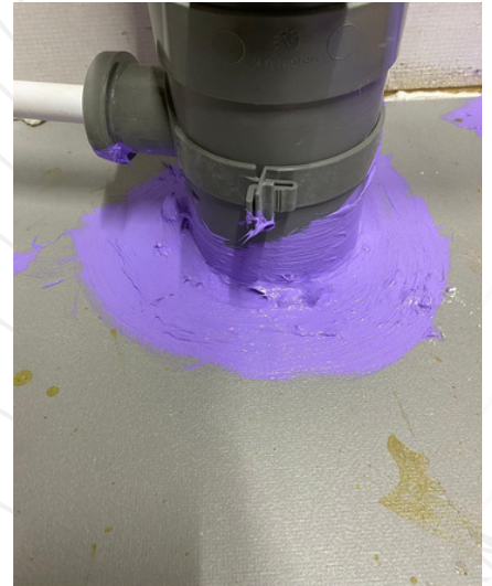
5.1.4 Soil stack through floor
