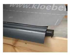
3. Lay the underlay so that it is level with the lip of the Underlay Support Tray, ensuring that it is not exposed to sunlight. Batten and tile as normal.
