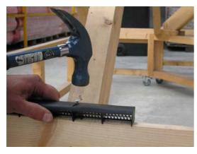
1. Set the fascia 30mm lower than normal. Fix the Fascia Vents continuously along the fascia.
