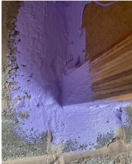
5.1.2 Joist connection into masonry wall
