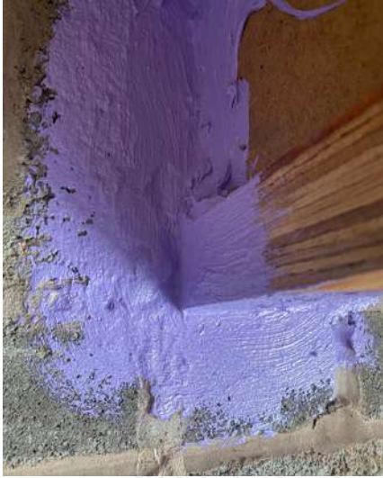
5.1.2 Joist connection into masonry wall
