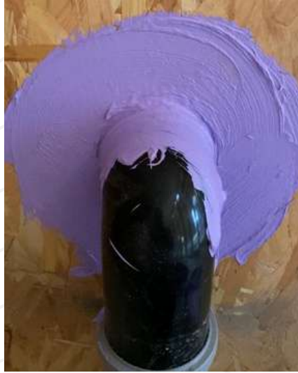
5.1.3 Pipe connection through timber frame
