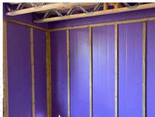
5.2.2 Service battens installed over Passive Purple Internal
