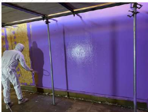
5.2.1 Spraying on to OSB board
