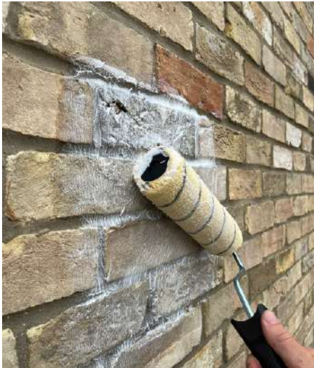
5.1.2 Roll applied Passivhaus Brick Seal
