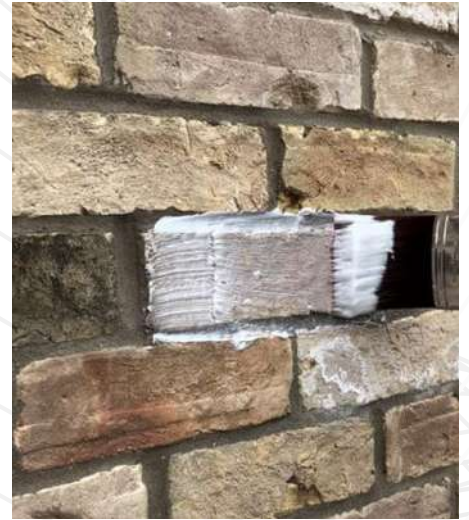
5.1.4 Brush applied Passivhaus Brick Seal
