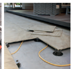
ON A RAISED OR PEDESTAL SYSTEM
