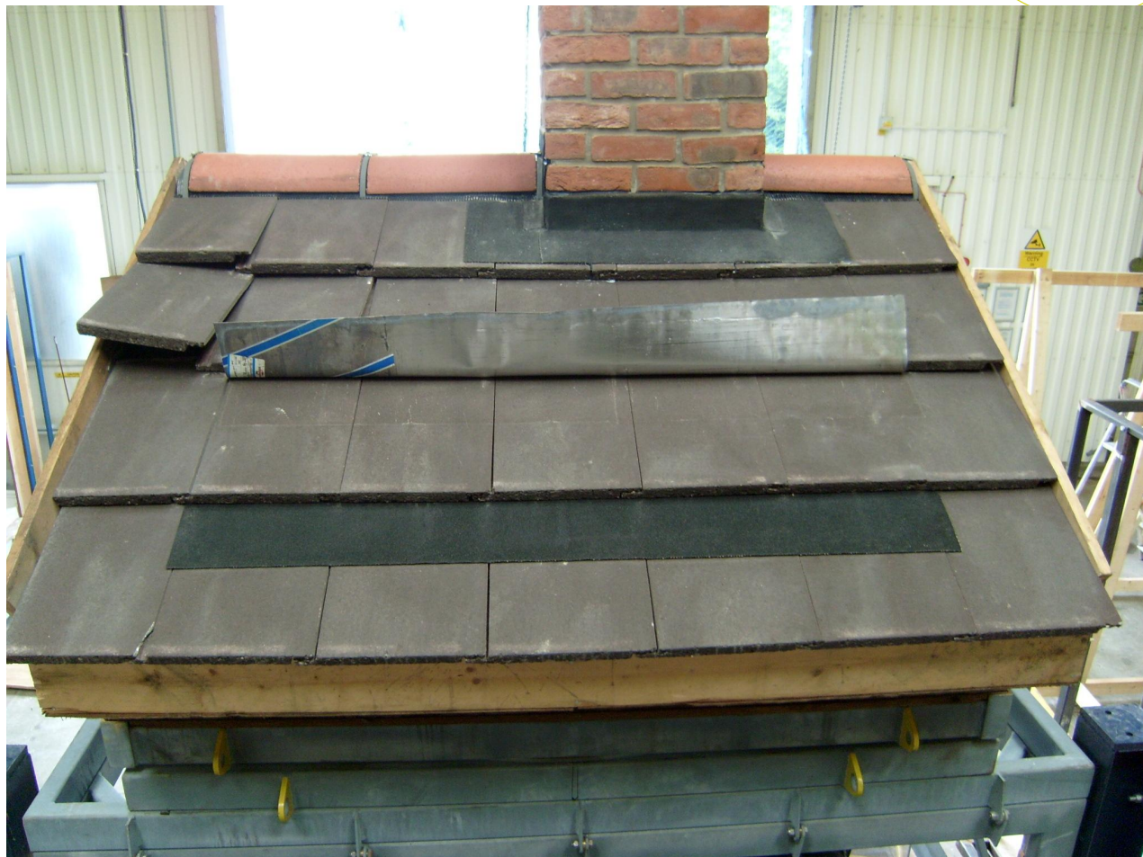
Figure A2 side 2 after completed test programme showing damage to lead flashing and tiles 45m/s (101mph)
