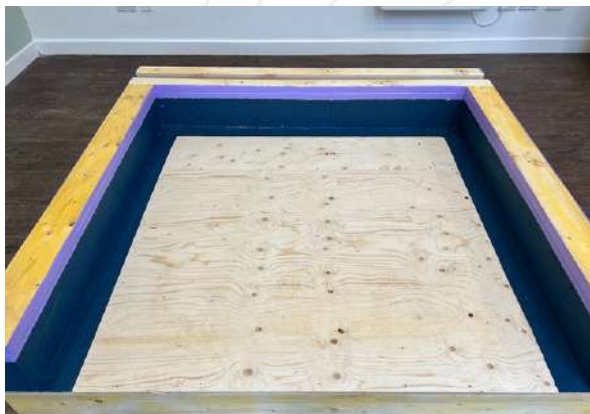
5.1.2 Timber frame, kicker block, and sole plate
