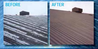
METAL-KOTE colour matched to original plastic coated profile metal roofs. which were flaking and peeling.
