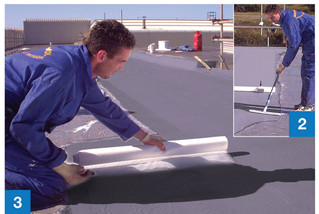
Pic 2. Apply an adhesive coat of Acrypol System 10 Undercoat at a coverage of 0.5 kg / m 2 - 0.75 kg / m 2 depending on surface porosity. Pic 3. Into this wet coat, incorporate Acrypol (1 metre wide), scrim and smooth flat.
