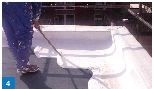
Pic 4. Apply Acrypol System 10 top coat. See reverse - Point 7 - for coverage information.
