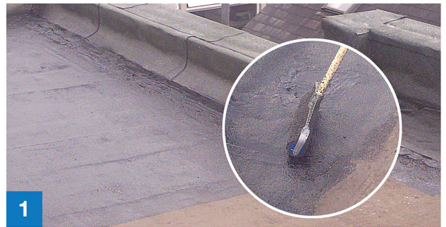
Pic 1. Apply Acrypol Sealer at a coverage of 6 - 8 m 2 / Ltr
