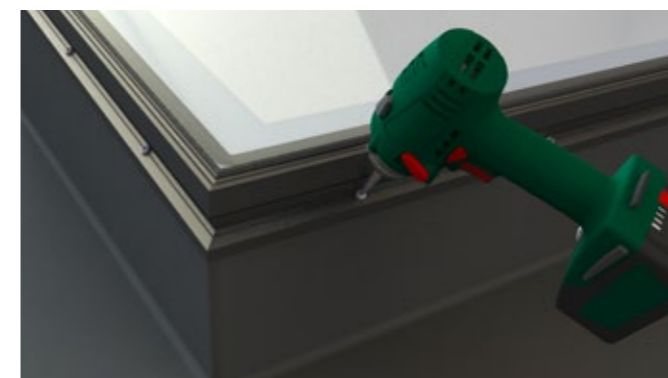
3 Screw the Rooflight onto the kerb using appropriate fixings. Secure it 150mm from the ends and 250mm centres.
