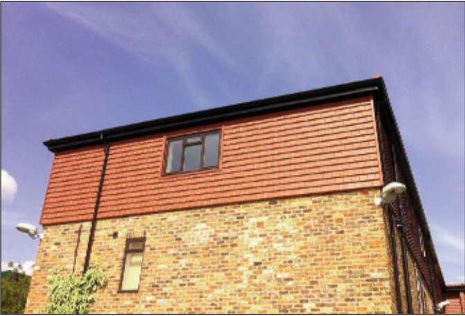
The plaintile's aesthetic characteristics and lightweight properties enable it to be used on a wide variety of applications, including vertical cladding.
