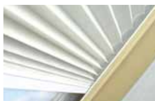
Side aluminium guides limit the amount of incoming sunlight
