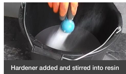
Thorough stir before decanting
