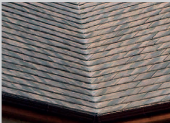
Hardrow® Slates Duets® Twilight roof incorporating purpose made valley.
