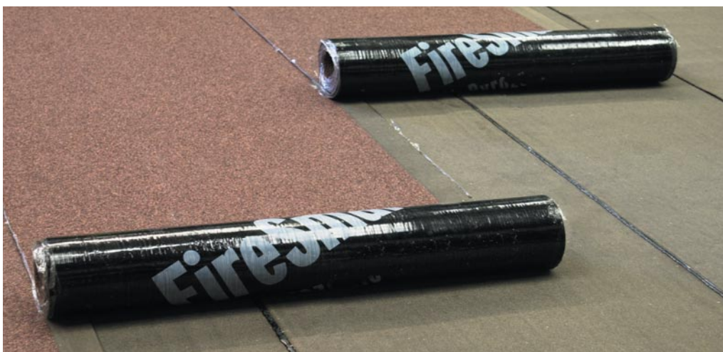
3. Setting out Cap Sheet offset 500mm.
