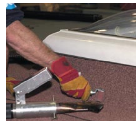
Positioning of supplementary Mechanical Fasteners if required.
