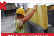
Do not push insulation down into the cavity as a tightly butted horizontal joint cannot be ensured.
