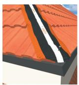
Starting at the eaves, centre the Roll-Fix® over the hip batten and secure using corrosion resistant nails or staples. Fix at 300mm centres along the ridge.
