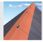
At the ends of the ridgeline, a clay plain angle block end ridge tile is recommended, which must be mechanically fixed into the ridge batten. A fixing hole will need to be drilled into the end of the ridge tile to allow it to be fully secured into the ridge batten.
