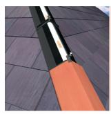
In principle the procedure for laying and fixing Roll-Fix  $^{\!\scriptscriptstyle (\!R\!)}$  with Clay Plain Hip Tiles on a slate roof is the same as for the fixing of concrete tiles. An exception to this rule is that a single 25mm ridge batten may be sufficient for some steeper angle Clay Plain Hip Tiles.
