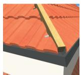
Commence tiling as normal, cutting tiles neatly along the line of the hip batten, making sure no cut tile is more than 30mm from the hip batten.
