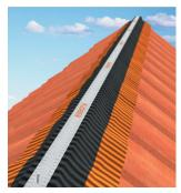
Starting at one case, and the Roll-Fix® centrally over Starting at one end, unroll the ridge batten, making sure there is 75mm cover each side of the top course of tiles. Secure in place using corrosion resistant nails or staples at 300mm centres through the white spine of the Roll-Fix®.
