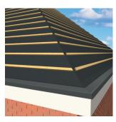
The roof underlay is laid in the normal way, making sure the tiling battens are secured directly onto the hip rafter or to noggins fixed to the side of the hip rafter in between the jack rafters. (This needs to be carried out before the underlay is laid).
