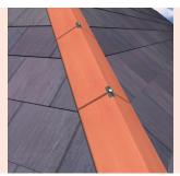
At the eaves junction at the base of the hip, a clay plain angle block end hip tile is recommended, which must be mechanically fixed into the hip batten.
