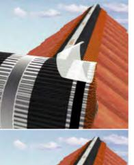
**5** Starting at one end, unroll the Roll-Fix<sup>®</sup> centrally over the ridge batten, making sure there is 75mm cover each side of the top course of tiles. Secure in place using corrosion resistant nails or staples at 300mm centres through the white spine of the Roll-Fix<sup>®</sup>.
