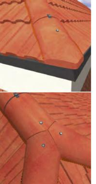
Secure the block-end hip tile to the hip batten using the 90mm screw and washer provided. Insert hip seals in between hip tiles and fix using the 90mm screw, washer and clamping plate provided. Continue this process up to the apex.
