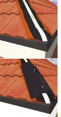
5 Starting at the eaves, centre the Roll-Fix® over the hip batten and secure using corrosion resistant nails or staples. Fix at 300mm centres along the ridge. Remove release paper from the adhesive strip and dress neatly, in a straight line, onto the dry, clean and dust-free tile surface. Continue up to the apex and onto the ridge batten. Note that the Roll-Fix® on the ridge needs to be lapped over the Roll-Fix on both hips.
