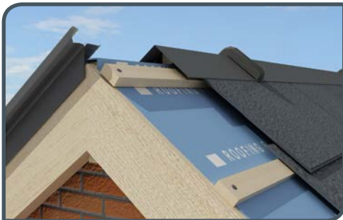
Fig.8. Nail L/H trim in place
