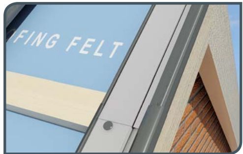
Fig.5. Insert upslope trim into lower trim section.
