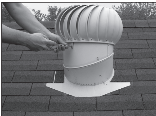
5. Insert a screw through the bracket hole into the new hole in the base and tighten. 6. Similarly drill and place the two remaining screws in the two remaining brackets.
