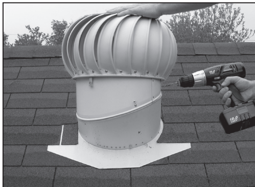
3. Set down gently until brackets on the inside of the turbine head contacts the top edge of the existing base. CAUTION: DO NOT TRY TO MAKE EXISTING HOLES IN BASE MATCH HOLES IN BRACKETS. THREE NEW HOLES WILL NEED TO BE DRILLED. 4. Using 1/8 drill bit, drill one hole through the base using the pre-drilled hole in the turbine bracket as a guide.
