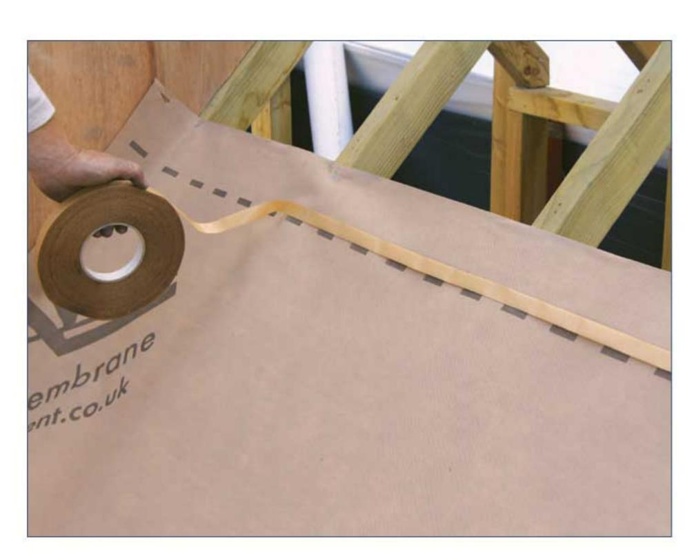
9. Install the next course with at least 150mm lap below a 25 degree pitch. Remove the covering layer from the tape and allow the top lap to stick to the tape.
