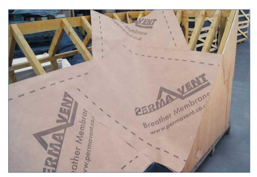
8. Permavent double-sided tape should be applied along the lap line before moving up to the next course. The tape can be pressed onto each rafter and it will naturally stick between the rafters. Taping the laps will also eliminate the rare occasions when wind driven rain can be forced under the laps if the roof is not covered in.
