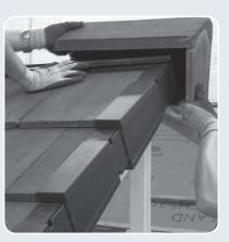
**7.** On gable end roofs, use left-hand and/ or right-hand Block-End Monoridge Tiles or Monoridge End Caps (LH/RH). Cut Monoridge Tiles should not be less than half their original length and should not be fixed within 450mm of the end of a ridge line. Carefully drill a 6mm diameter hole, 30mm in from the end of cut Monoridge Tiles. When using Cloaked Verge at the left-hand verge, cut a Profile Filler Unit to fill the open end.
