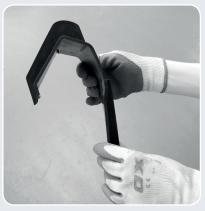
5. Fold leg of Ridge-to-Ridge Seal and slide under the open end of the first and subsequent Monoridge Tiles.
