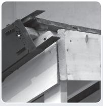
**3.** Fix a 25mm thick continuous ridge batten to the back of the rafters. Lay and fix tiles in accordance with manufacturers fixing specification.
