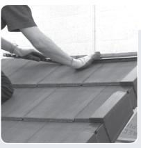
4. Lay Profile Filler Units along the roof tiles snapping them together so they are ready to accept the Monoridge Tiles. If necessary, cut the filler unit to suit the ridge length.
