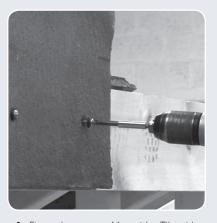
6. Fix each concrete Monoridge Tile with two woodscrews and neoprene washers supplied, screwing into the continuous ridge batten. Slide the next Monoridge Tile over the Ridge-to-Ridge Seal. Continue laying and fixing Monoridge Tiles and DryVent Monoridge components along the ridge line.
