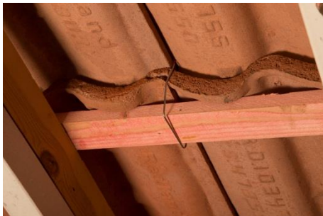
Figure 9 – Innofix Clip installation instructions
