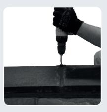
STEP 7. MECHANICALLY FIX THE TILE Insert the woodscrew through the clamping plate and either embed it into the mortar joint between the tiles or insert it through a pre-drilled hole in the centre of the ridge tile. Screw the woodscrew in ensuring that it remains perpendicular to the roof.
