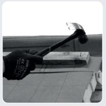
STEP 4. COVERTHE RIDGE / HIPTREE Cover the ridge / hip tree with underlay and fix the top tiling batten in the usual way.
