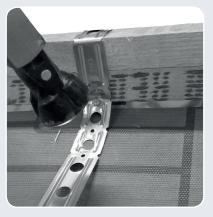
STEP 3. FITTHE BATTEN STRAP Position the ridge batten along the centreline of the apex. Nail the Batten Straps to the rafters using two  $30\times2.65$ mm annular ring shank nails provided.
