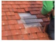
26 Continue to replace all the remaining tiles, checking that they're all sited properly before leaving the roof.
