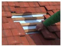
**5** Cut along the marked lines. Two of the three tiles will need their corners removed.
