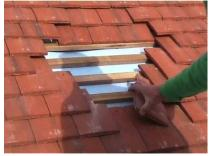
9 Cut through the two battens along the marks and remove the centre sections. Now assemble the ducting.
