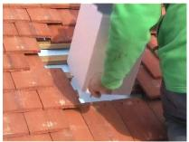
13 Using a sharp bladed knife cut diagonally from corner to corner in an x shape through the felt, creating four triangles. Return the ducting and push it down through the cut felt to rest on the plasterboard ceiling below. Make sure that the ducting is square and perpendicular to the tiles.
