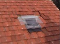
21 Replace the three bottom tiles you cut earlier by carefully sliding them under the bottom edge of the Suntile and over the black, under tile gasket.
