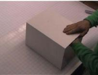
11 Cut the Silver Tape to the length of the joint, remove the backing tape and stick over the jigsaw joint. Smooth the tape down on the top surface and then flip the duct over and push firmly down from the inside along the jigsaw edge to make sure the edges are all in firm contact with the tape.
