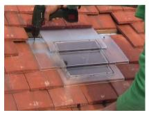
25 Start replacing the remaining tiles by sliding up underneath and locating them onto the battens.
