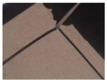
15 Return to the inside of the property. Take the ceiling template provided and push the bradawl though the top left hand corner at the mark "Suntile Basic Kit Ceiling Holes". Push the bradawl through the hole made in the plasterboard earlier and pivot the template until perpendicular. Hold the ceiling template firmly in position and draw around the template's outside edges.
