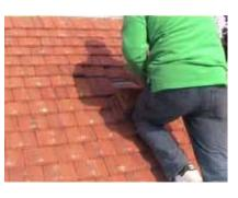
2 After removing the marked and overlapping tiles, return the Suntile to it's proposed position. You will notice that the Suntile's square box flange sits on top of three tiles along the base.
