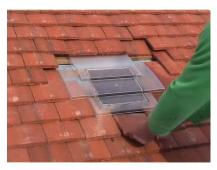
22 Detach the three tile retaining clips from the "u" shaped component taken from the black under tile gasket.
