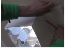
28 Cut all around the ducting using a sharp blade along the offset line and remove the waste.
