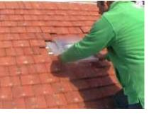
3 Mark the three tiles around the bottom and sides of the Suntile flange. Then remove the Suntile.
