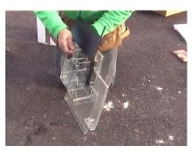
19 Push the mirrored duct inside the Suntile's square box flange, make sure the ducting slides down to touch the clear surface. Use the silver tape to cover the joint between the ducting and the flange in one continuous length, smoothing the tape firmly into the joint and the corners, finally cutting the tape to allow an overlapping joint. We recommend that a second and third wrap of silver tape should be carried out overlapping the first taping top and bottom.
