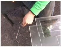
**18** Connect the gasket to the Suntile's square box flange by sliding into the three slots on the flange as shown. Push the gasket firmly down towards the Suntile's top surface, until it should come to a stop about 20mm from the underside of the Suntile. Make sure the gasket runs perpendicular to the surface of the Suntile.
