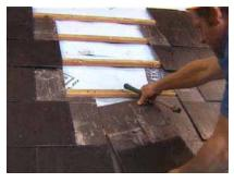
3 Cut the slate along the marked line with a disc cutter. Cut through the batten where you marked it.
