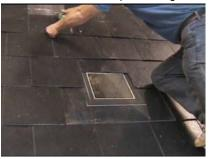
20 Back inside the ducting now needs to be trimmed to take the ceiling diffuser assembly. Use a 6mm thick piece of flat material as a spacer to mark a 6mm offset line around the outside of the ducting parallel to the ceiling. We used a small piece of 6mm thick cardboard.
