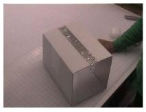
10 Push the assembled ducting inside the flange on the underside of the Slate Suntile; make sure the ducting slides down to touch the clear surface. Use the silver tape to cover the joint between the ducting and the flange in one continuous length, smoothing the tape firmly into the joint and the corners, finally cutting the tape to allow an overlapping joint. We recommend that a second and third wrap of silver tape should be carried out overlapping the first taping top and bottom.
