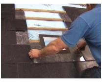
**5** Measure the distance from the top of the cut slate to the top of the Suntile's flange. Remove the Suntile and mark the position of the Suntile's top flange edge onto the felt .
