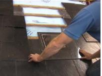
**16** Screw the Suntile to the battens through the holes provided. Then start to replace the original slates working from the bottom to the top, left to right.
