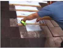
**6** Using a sharp blade knife, cut through the felt corner to corner in an X shape creating an aperture to fit the flange on the Suntile.
