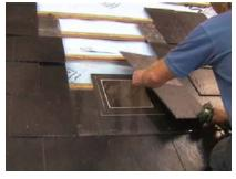
17 Fix with screws as necessary. Stop when you reach the centre slate that would cover the Suntile's lens.
