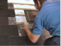
12 Remove the Suntile & ducting, take a bradawl and push a hole through the plasterboard ceiling in the top right hand corner
