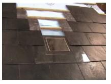
18 Position the centre slate just above the lens area of the Suntile and mark the top edge in line with the slates either side of it. Cut the slate along the marked line with a disc cutter.
