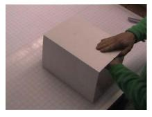
**9** Cut the Silver Tape to the length of the joint, remove the backing tape and stick over the jigsaw joint. Smooth the tape down on the top surface and then flip the duct over and push firmly down from the inside along the jigsaw edge to make sure the edges are all in firm contact with the tape.
