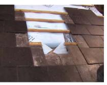
7 Trim off each of the four, felt, triangular shaped flaps, leaving a clear, square aperture. Refer to the ducting assembly instruction provided, i.e. points 8, 9 and 10, and assemble the ducting including taping the ducting to the Suntile. Reposition the tile with the ducting in place.
