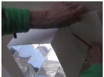
21 Cut all around the ducting using a sharp blade along the offset line
