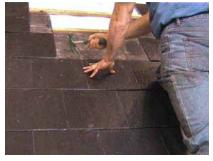
2 Once you have removed all the necessary slates down to the bottom edge of the Suntile's final planned position as shown, place the Suntile into position and mark the slate along the bottom edge of the Suntile's flange and also where the flange passes over the exposed batten. Remove that slate for cutting.
