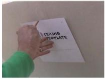
14 With a sharp knife or grip blade cut along your drawn lines and remove the plasterboard square.
