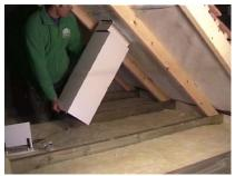
11 In one continuous strip carefully tape the joint between the two parts, making sure the tape is firmly smoothed down. We advise that you tape around the joint three times, overlapping the first tape top and bottom. Once secure you can gently bend the duct, as previously shown, into alignment with the ceiling. The duct should finish between 50mm – 250mm from the plasterboard ceiling level. It can be easily cut with a sharp bladed knife as before.
