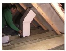
12 Using a bradawl push a hole through the plasterboard ceiling in the bottom left hand corner of the duct, where the ducting would touch the ceiling. See X in above right photo.
