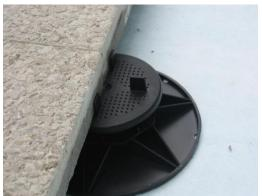
For decks built to a larger fall SLOPE CORRECTORS can be fitted to the base plate to create a level surface.
