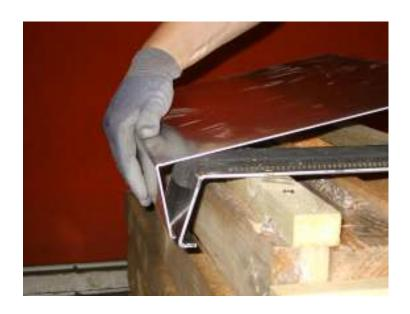
Locate wall coping over half of the wall bracket at joint and rotate down.
