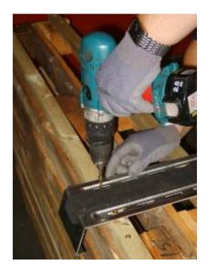
Insure that a minimum 31mm gap is left on the overhang.
