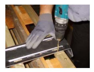
Using recommended fixing screws, fix wall coping strap to structure at maximum 1.5metre centres or as recommended based on wind uplift calculations. Note. water proofing membrane by others not shown.
