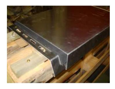
Apply pressure to the coping so as to clip the coping in place. Compressing the EPDM seal as shown. Repeat on the next length or fitting. Leave 4mm gap for expansion
