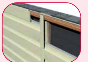
fig 11 Top edge detail showing packing piece and 2-part Universal trim.
