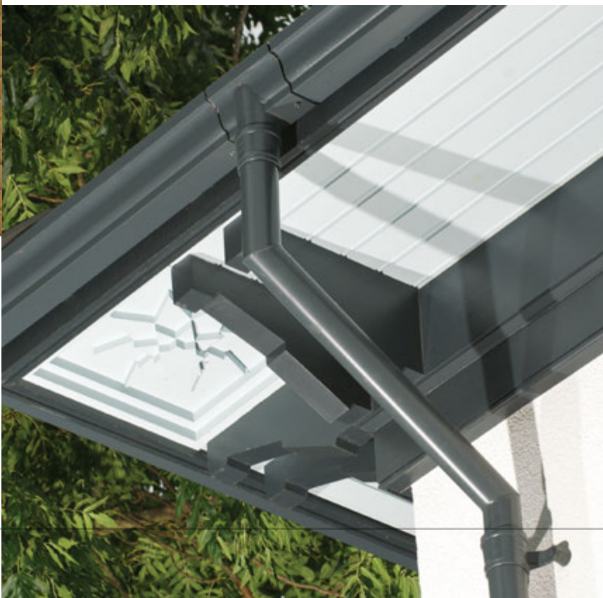
Prince's Foundation Natural House, BRE, Watford
