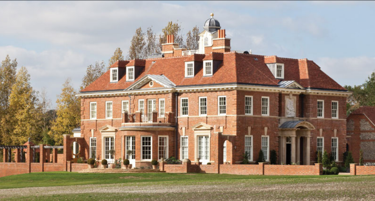
Prestige new build, Hampshire
