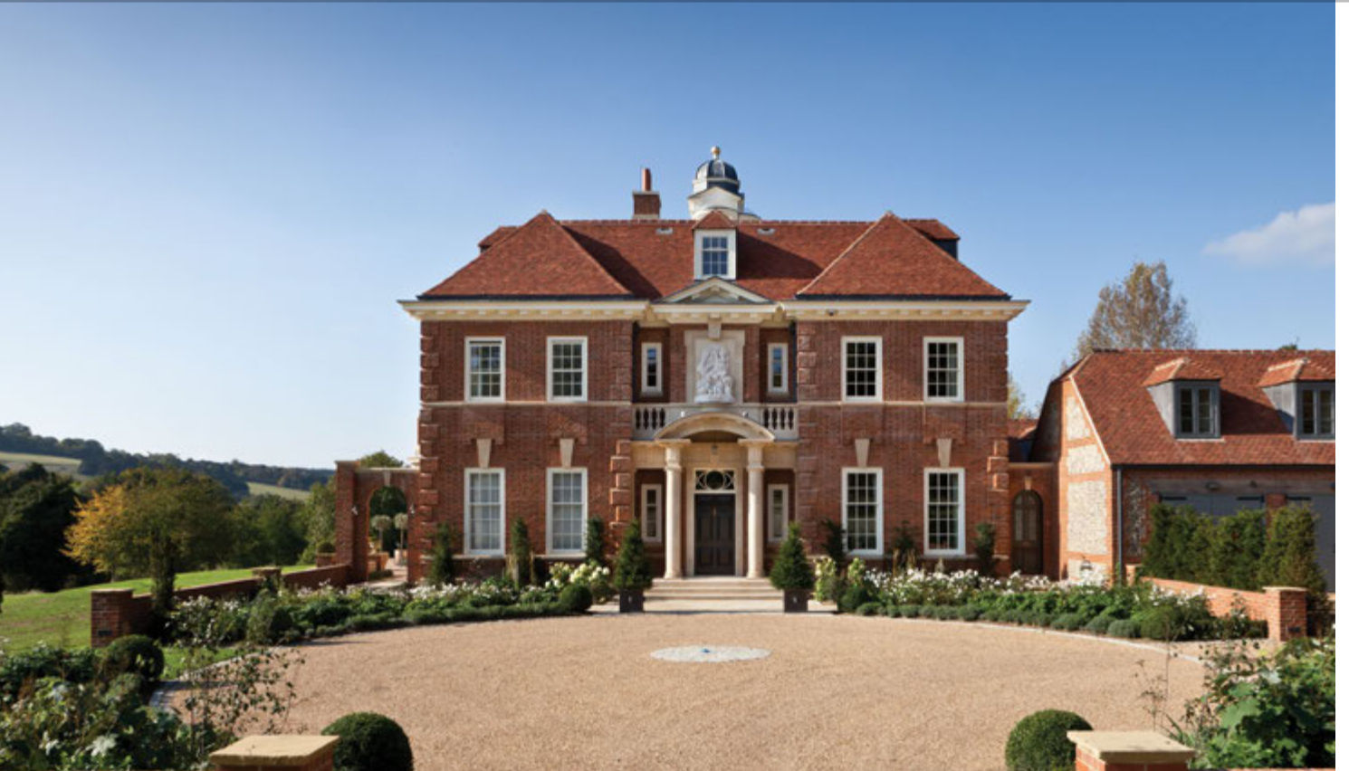
Prestige new build, Hampshire
