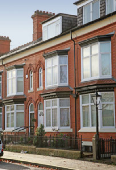
Social Housing refurbishment, Manchester
