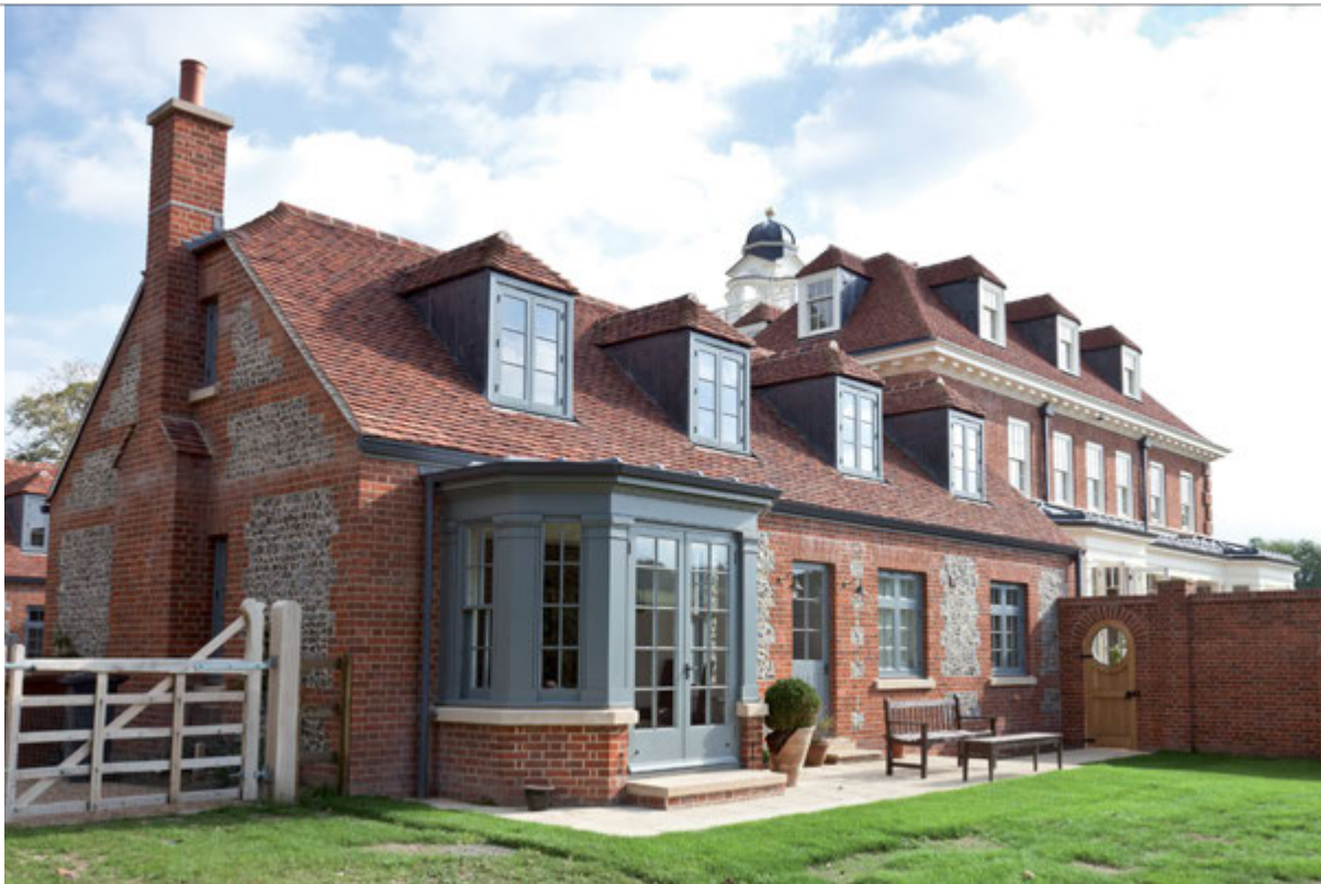
Prestige new build, Hampshire
