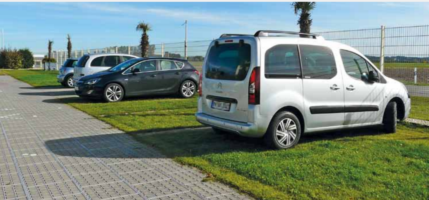
Sustainable and durable: TTE® parking spaces and driving tracks after being used daily for 10 years (TTE® Construction Principle 1).
