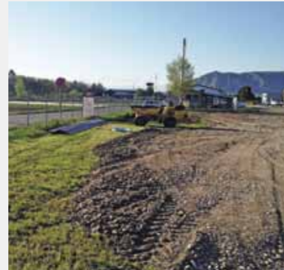
Application and distribution of the gravel sand mixture directly onto the existing top soil
