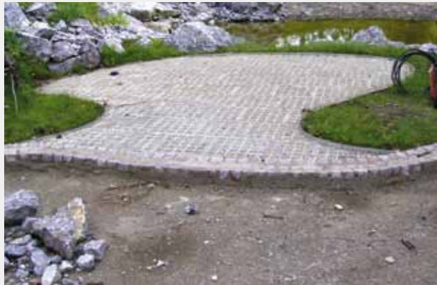
Laid and filled TTE® elements BEFORE installation of the water-bound covering.
