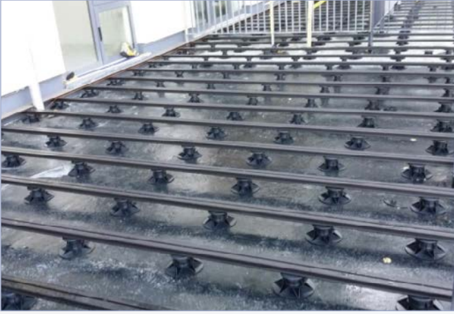
Flat Headed Pedestals can be used with larger timber joists or the aluminium rails available as part of iDecking EasyClick system, available exclusively through Wallbarn.
