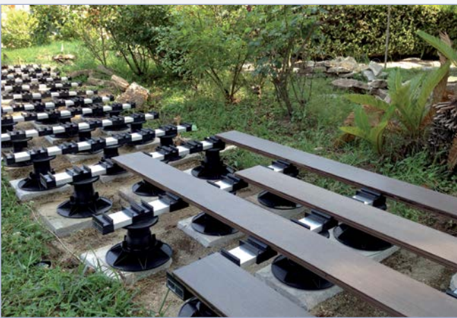
Flat Headed Pedestals can be used with larger timber joists or the aluminium rails available as part of iDecking EasyClick system, available exclusively through Wallbarn.
