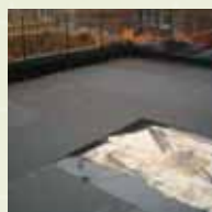
Protecto-board – bituminous protection membrane to prevent punctures and abrasion to bituminous waterproofing
