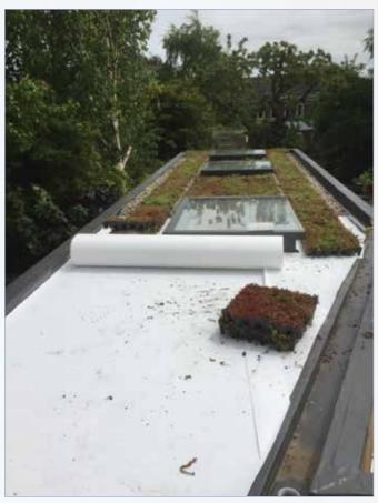
A separation and filtration geotexile layer should be firstly installed onto the deck. This protects the waterproofing and prevents abrasive damage. Wallbarn usually can supply a 300gsm recycled fleece for this purpose as an additional item.
