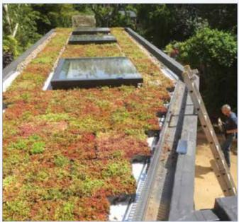
The edges should be filled with a border of washed riverstones, in accordance with the GRO code of practice. Objects such as roof lights and cables should be surrounded with riverstones to prevent root invasion and act as a fire break.
