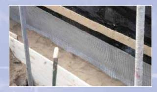
As the water drains vertically down the membrane, it should be channelled into a perforated pipe. The geotextile fabric can be pulled away from the HDPE membrane at the bottom of the structure to wrap
