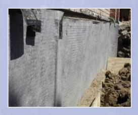
Protecto-drain G8 is suitable for areas with a much greater amount of water passage and pressure through the ground.
