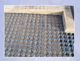
For INTENSIVE green roofs installers will need to use Wallbarn Protecto-drain 60P as the drainage membrane.
