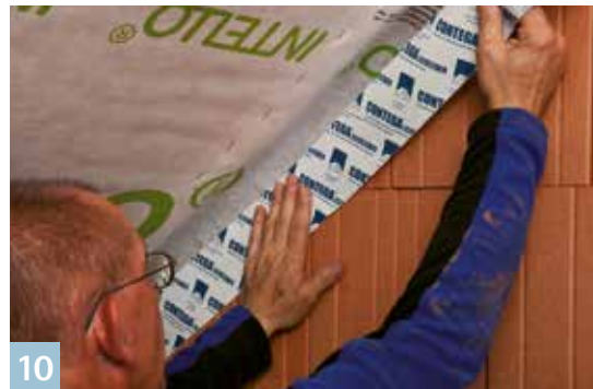
CONTEGA PV Plaster sealing tape for defined, permanent, reliable joints with substraces that are to be plastered
