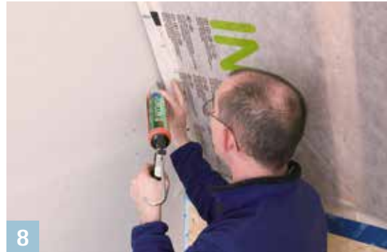
ORCON F System adhesive for bonding to adjacent components
