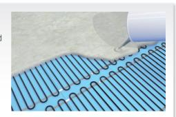
If you are using a suitable vinyl/ carpet or engineered/laminate floor as the final covering then we recommend a minimum of 8mm suitable latex levelling compound to cover the heating mat/cables to ensure even heat distribution.
