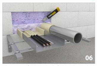
• Cut any excess foam away. Cut the foam away up to a depth of 4mm across the whole surface along both sides of the opening. Use a sturdy knife.
