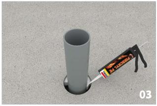
• Apply Firecryl FR around the pipe on both sides of the opening.
