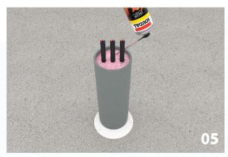
• Apply Soudafoam FR between the cables in the PVC pipe.
