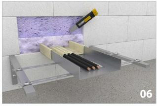
• Cut any excess foam away. Cut the foam away up to a depth of 4mm across the whole surface along both sides of the opening. Use a sturdy knife.
