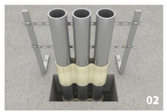
• Put the cables in the cable duct.
