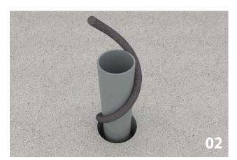
• Apply a PU joint filler around the PVC pipe for half the thickness of the ceiling.
