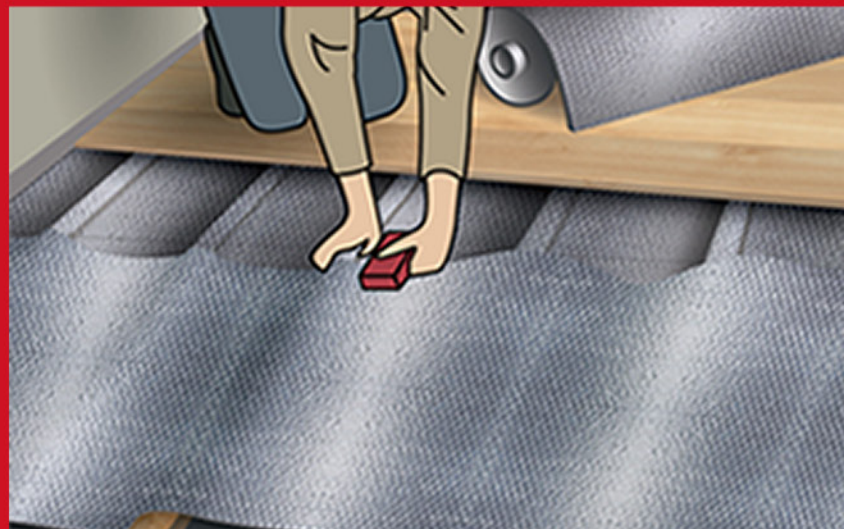
FLOOR APPLICATION - Equivalent to 60mm Mineral Wool
